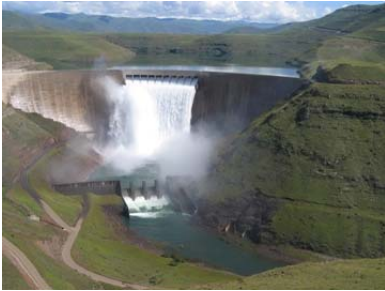
The dam is full to over flowing...like our blessings!
